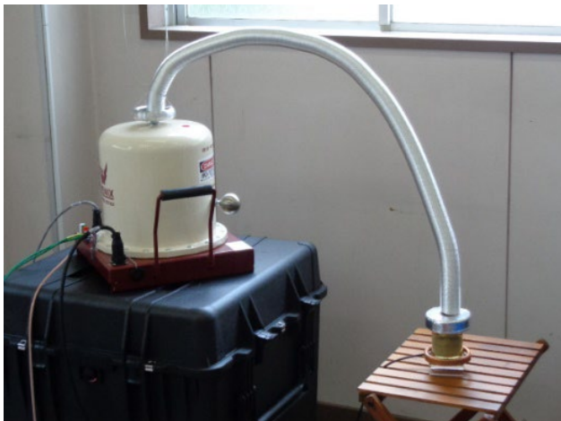
High voltage transformer (50 kVrms) and a partial discharge source.
